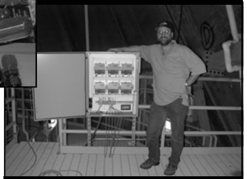
Glenn McNair with strobe controller power supplies during installation.
