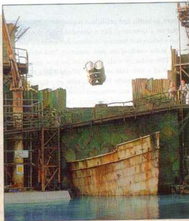
The "Pig" makes its first flight on the newly constructed set in Japan. Notice the tip of the launcher track visible through the cutaway section of wall. The hole will later be filled with breakaway foam sections. The permanent, themed crane arm on the left is used to reset the seaplane between shows.
