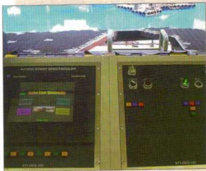
The main show console behind the audience overlooking the pool/stage. The primary effect-enable buttons for pyrotechnics, mechanical, and flame effects are duplicated beneath the technical director's left and right hands. The T-shaped arrangement of buttons controls the progress of the technical script that synchronizes the sound, lighting, effects, and other elements of the show. The touch-screen on the left displays current status as the show plays and is used between shows for manual operation and reset of equipment.
