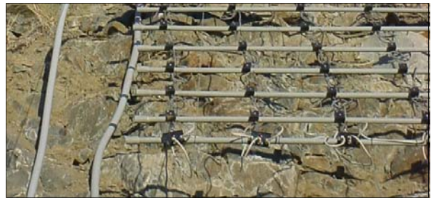
Close-up of LightNet deployed over the rocky surface.
